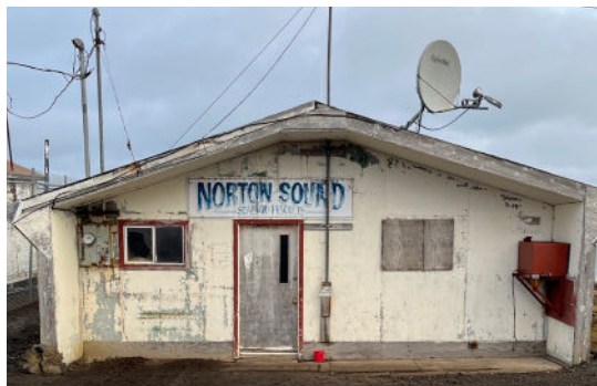
NSSP Seafood Plant facility in Savoonga on St. Lawrence Island.
