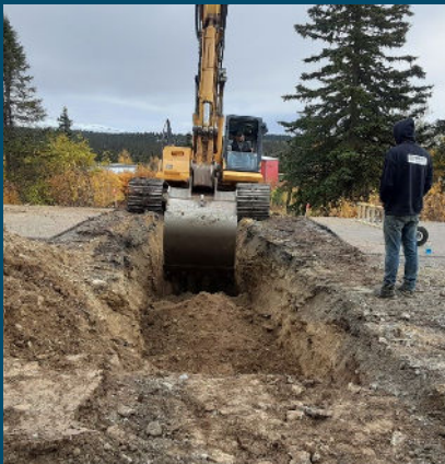
Breaking ground in Elim on water & sewer projects.
