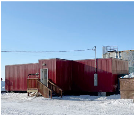
Recently completed Stebbins Washeteria Facility, supported in part by NSEDC Water & Sewer funding.
